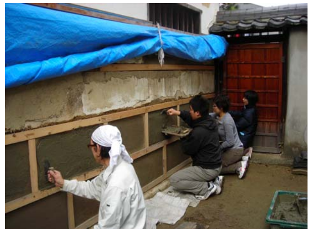
Earthen Wall Plastering at Naya Museum
