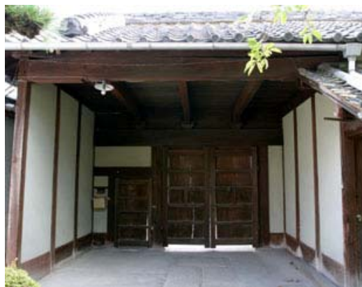
Photo 26 Stone terrace under the roof of the “nagayamon”(6 tatami mat size)
