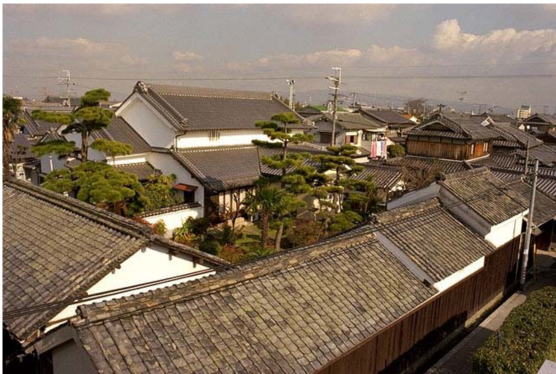
Photo 1: An Overall View of the Hatada-Family House
