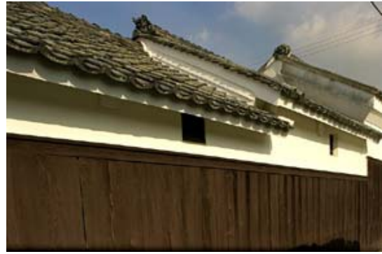
Photo 9 The east, central and west storehouse
