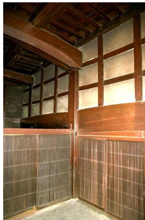
Photo 5: Massive structure of the beams above the “doma (earthen-floored area)”
