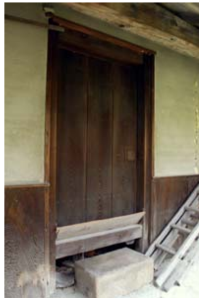
Photo 11: Door and Nezumi gaeshi (mice barriers) of the storehouse
